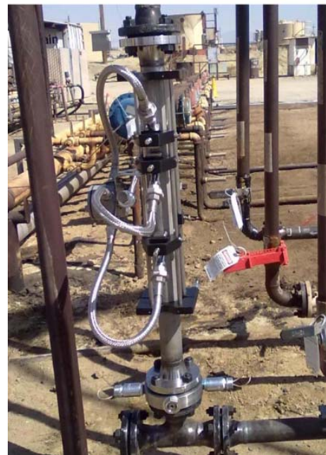
The Safire multiphase flowmeter undergoing extended testing
